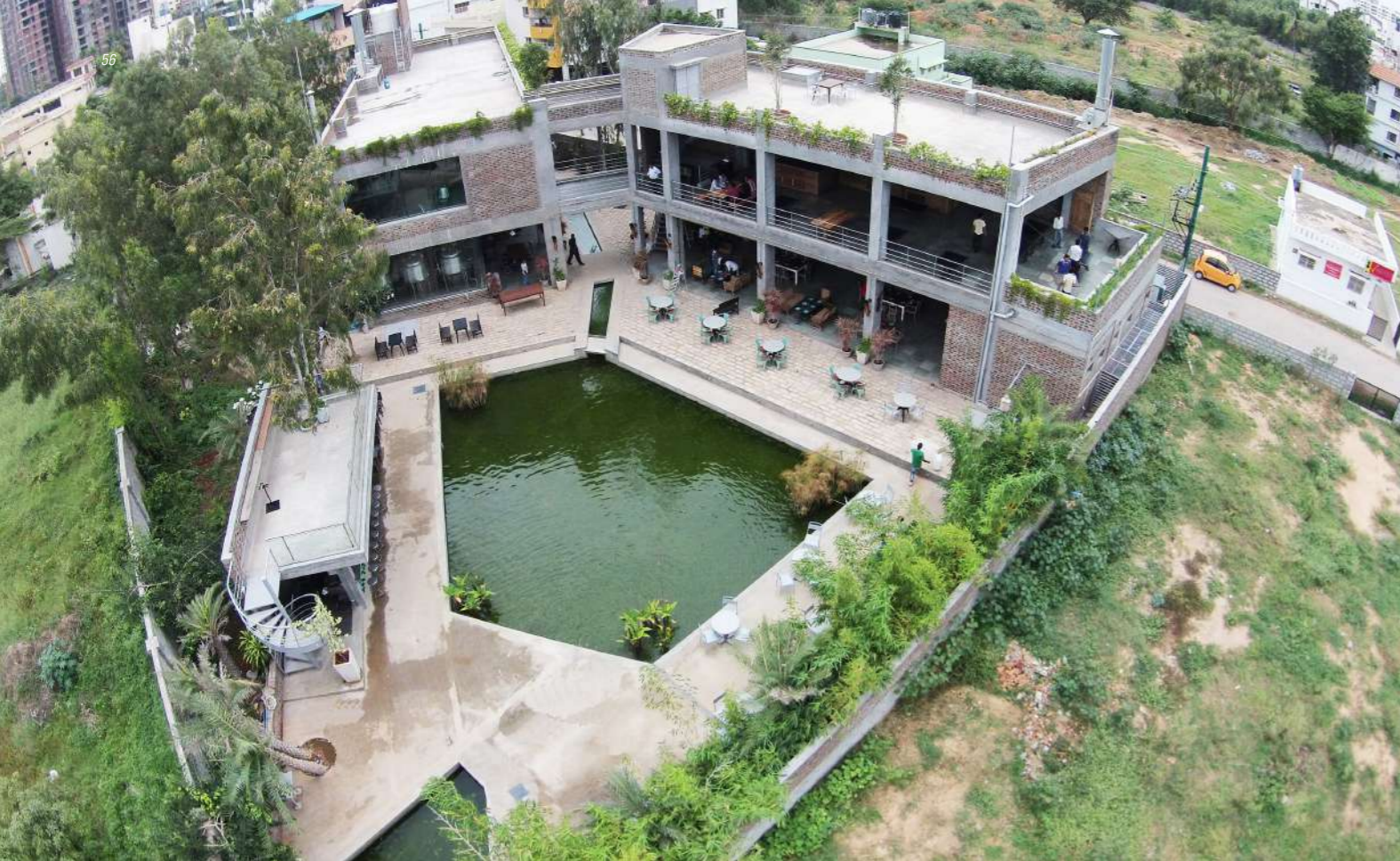
↑ View showing the courtyard, water body and outdoor seating.
